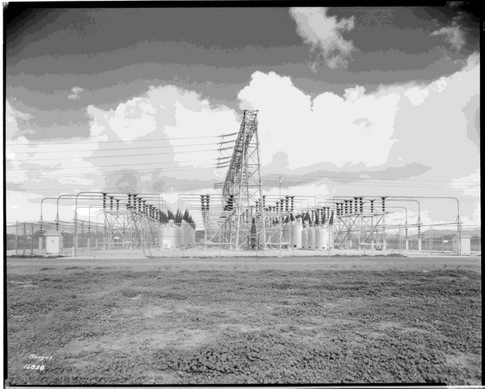
Image 8. Newly installed 220kV rack at Saugus Substation in 1930 (HDL Call No. 02-16898)
