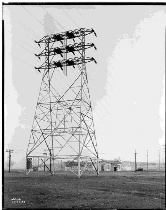
Image 6. Big Creek steel tower double-circuit at Saugus in December 1928 (HDL Call No. 02-18514)
