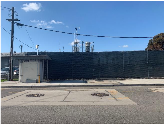
Figure 7 Street vault with manhole covers.
