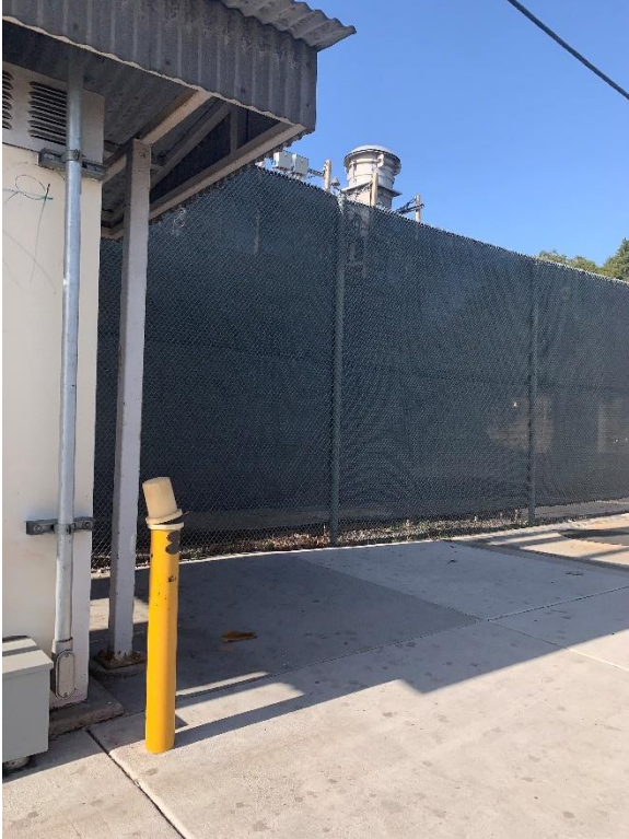
Figure 4 Tesoro Do Not Dig Post with Hudson Station in background.
