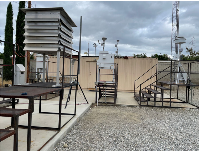
Looking at the probe from the South.
