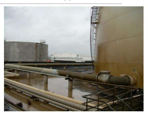
Open pipe channels designed for spill containment
