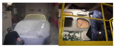
PREPARATION FOR PAINTING Be sure parts are free of grease, oil, rust or dirt. Sand and or grind remaining surface imperfection. Use clean cloth or solvent wipe to remove any residual smut or dirt. IS-279, Is-299,IS-300, IS-302 or acetone can be used for Zero VOC Surface Cleaners on many substrates. Remove any mildew with tetra-sodium phosphate and bleach; Correct surface defects; Seal surfaces that might cause staining through topcoat.
