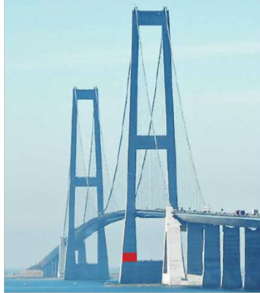
Figure 1 Automatic Sniffer measurements at the Great Belt bridge are conducted from the eastern Pylon (marked in red). Here 25000 ships are passing annually to reach or leave the Baltic Sea. Chalmers has measured more than 20,000 ships at this site since 2015 (Mellqvist 2018).
