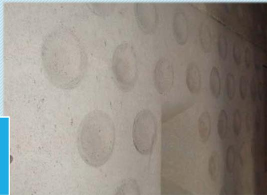
Patented dimple pattern Interior radiant wall
