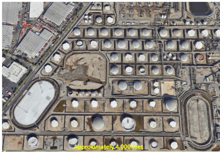
Figure 2.2 – Tank Farm at Rule 1178 Facility
