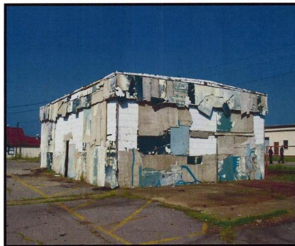
AACM2 building with added asbestos-containing Transite prior to demolition. (EPA photo)
