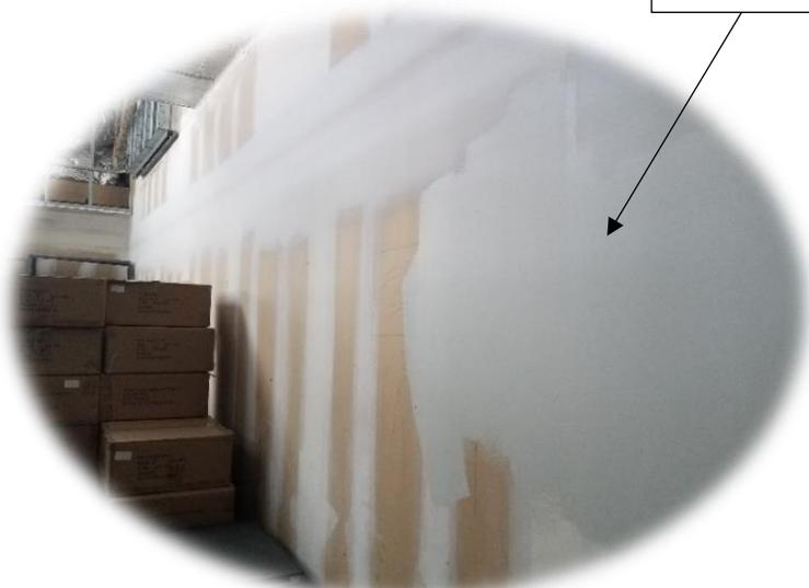
Figure 3: Photo of a partially painted wall system with paint (right side) covering joint compound and concealing where it was applied to the wall system
