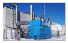
levels never approach the lower explosive limit and also maintains an optimal concentration for the catalytic bed to minimize required natural gas or electricity to maintain the optimal temperatures. The APCD systems were able to demonstrate control efficiencies between 99.95% to 99.99% through source testing.
