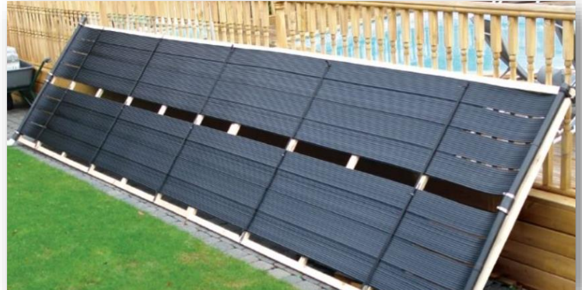
Solar in-ground swimming pool heater
