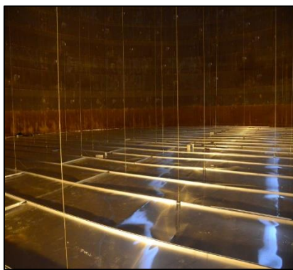
Figure 2-4: Cable Suspended Roof
