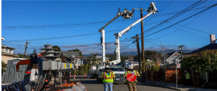
PG&E subcontractor crews install a new utility post in Oakland, December 2024.
