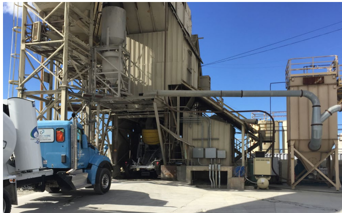
Concrete and Asphalt Manufacturing
