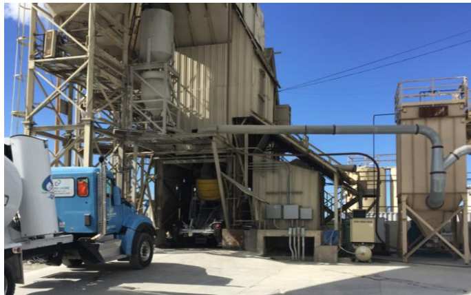
Concrete and Asphalt Manufacturing
