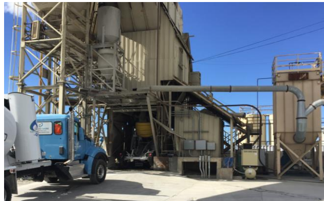
Concrete Batch Plants
