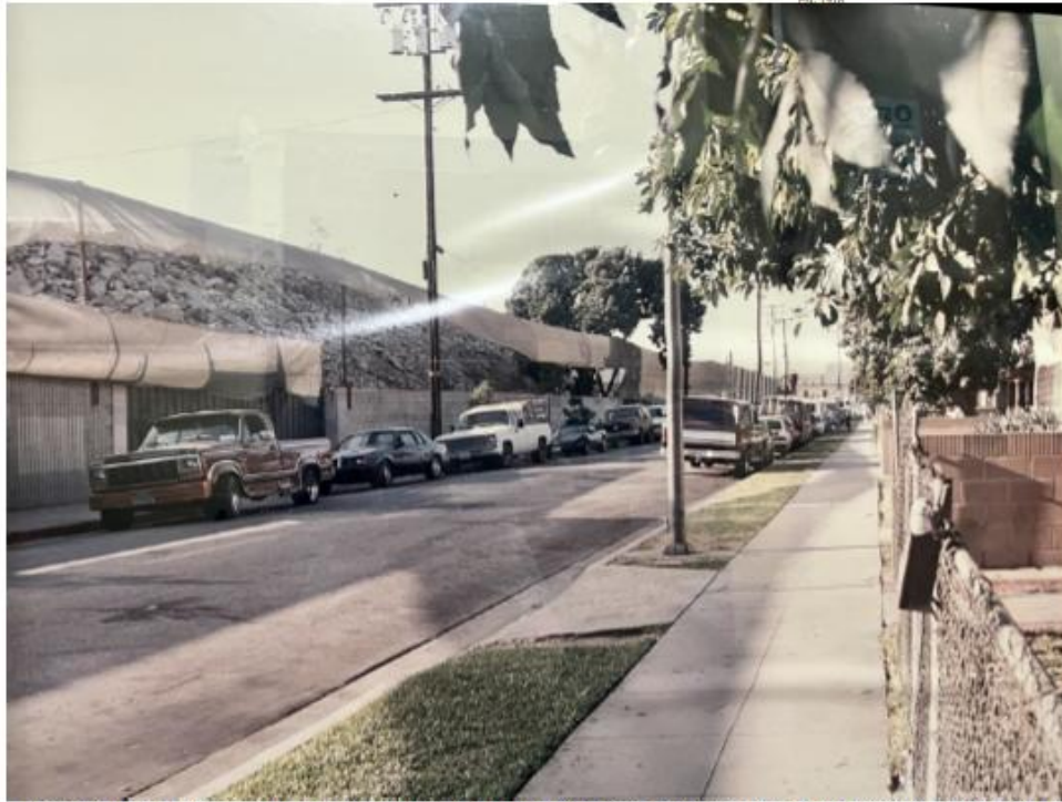
Figure 3: The wind screen fence surrounding La Montaña with gaps and tears. Residents had to live with dust and aggregate material spilling into their homes, cars, and public streets.
