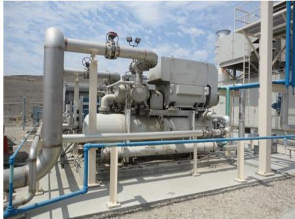
*Figure 27. Gas Compressors Arrangement*
