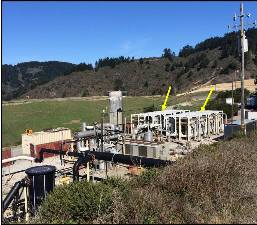
Figure 18. Overview of a Portion of the Gas Treatment System (arrows indicate the two eight-canister banks)
