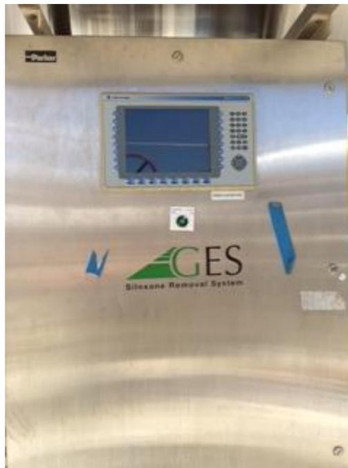
*Figure 24. Parker Siloxane Removal System Control Panel*
