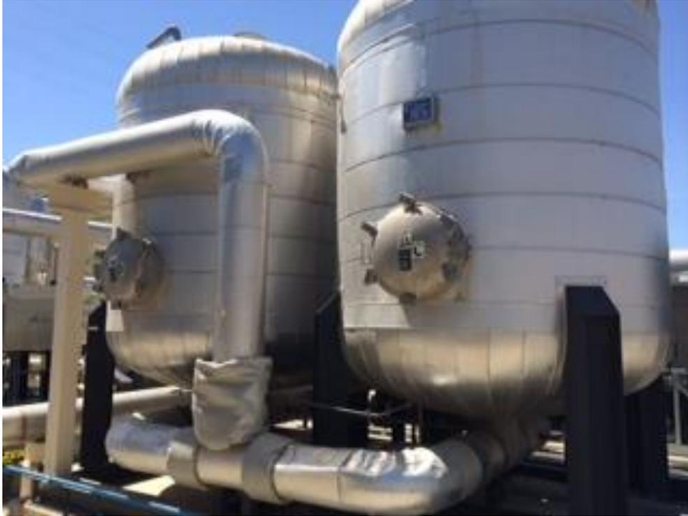
*Figure 23. General Setup of Vessels for the Siloxane Removal System
