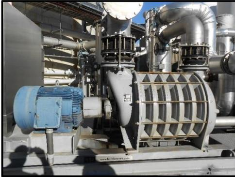
*Figure.13. Biogas Compressor at East Bay MUD*
