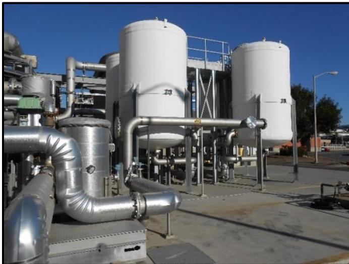
*Figure 14. Siloxane Canisters at East Bay MUD*
