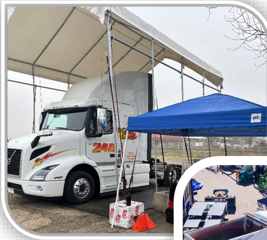
Site staging area at CSU Fresno (top left)
